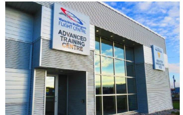
Hangar 7 Signage was installed January 2025
